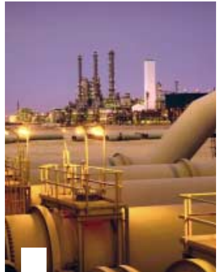
The ORYX GTL plant in Qatar will contribute towards Sasol's ongoing drive to develop and market fuels that are cleaner and more carbon-efficient.
