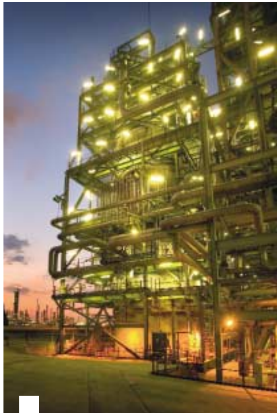
A Sasol Advanced Synthol™ (SAS™) reactor at Secunda lies at the heart of our Fischer-Tropsch coal-to-liquids (CTL) process.
