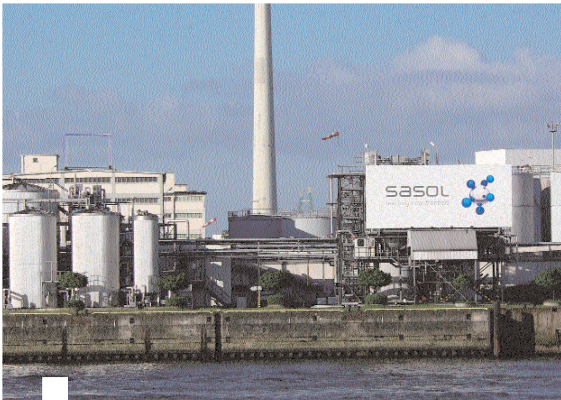
The Sasol Wax plant alongside the River Elbe at Hamburg, northern Germany. This business improved the performance of its steam-generation units and reduced carbon-dioxide emissions by 20%.
